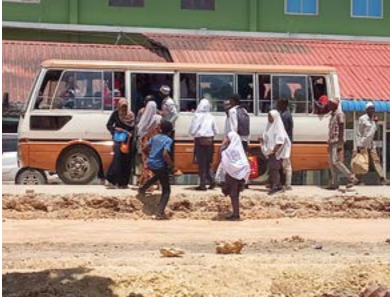
Above: A daladala stop for passengers. Below: Karume Road, Urban Unguja. February, 2024 Unguja, Zanzibar
